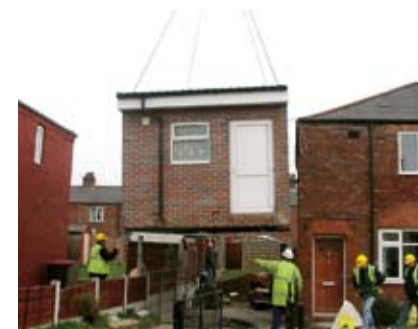
Relocatable factory-made modules offer a rapid means of providing disabled facilities at home
