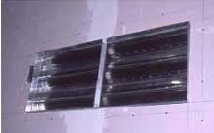
**Plate 8. Multi-blade damper mounted in Dry-lined partition**
