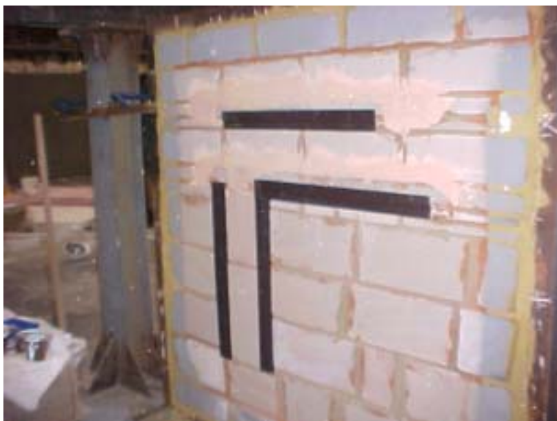
Photograph E9. Material installed in the test frame
