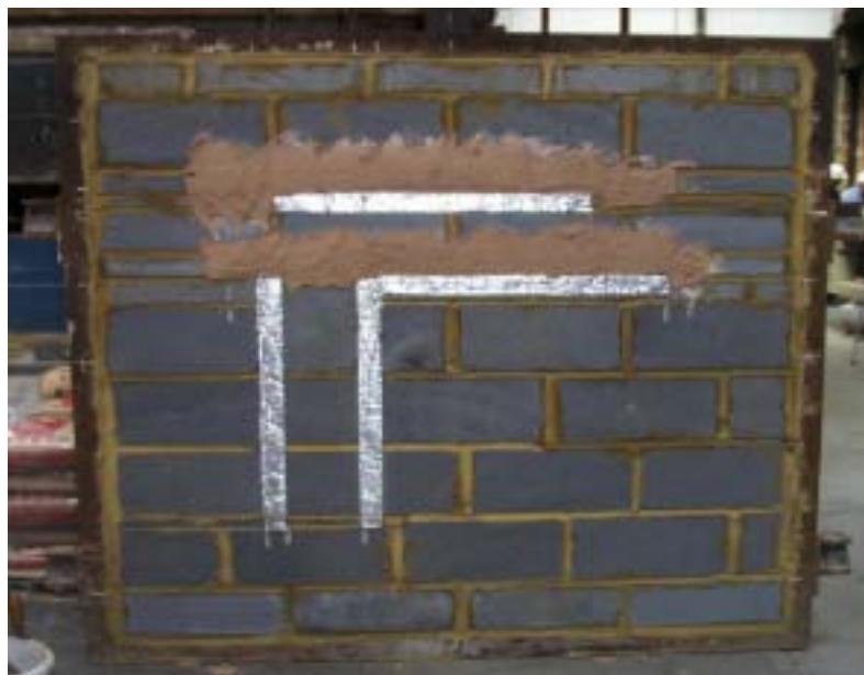
Photograph E3. Material for Test 1 installed in the test rig
