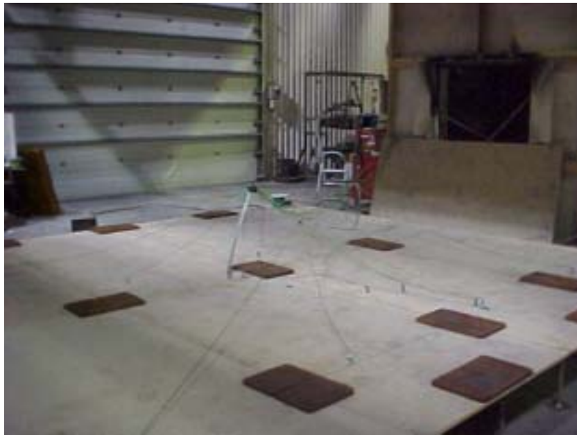
Photograph A3. Chipboard Floor.
