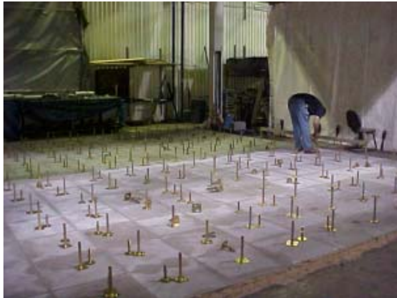
Photograph A1. Suspended floor under construction.
