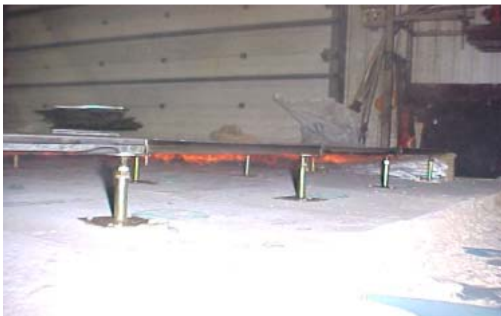
Photograph 14. flames impinging on the cavity barrier.
