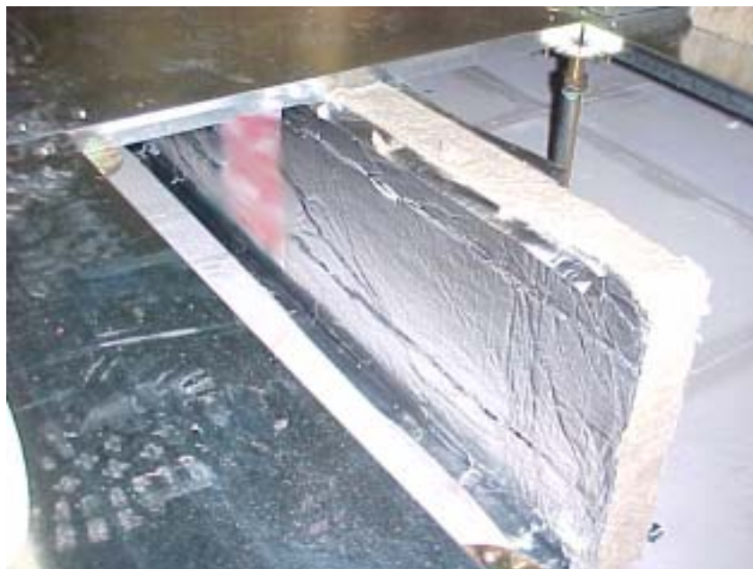
Photograph A2. Cavity barrier in floor void. (Tile removed)
