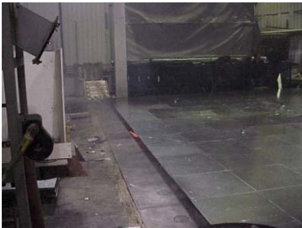
Photograph A13. Shows flames emerging from the edge of the floor.
