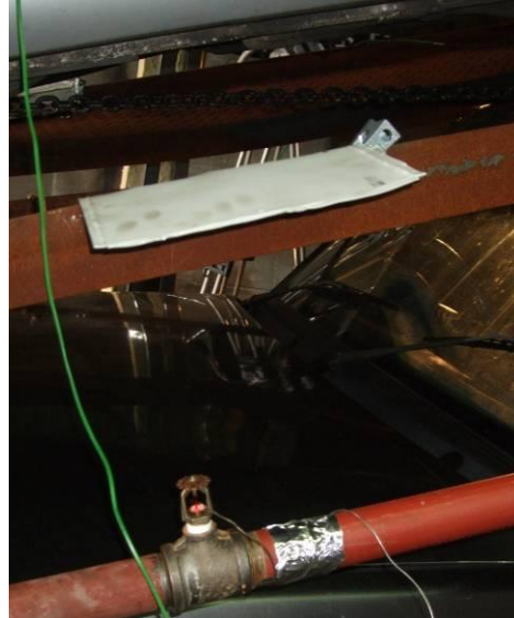
Figure 7 – Baffle plate installed above intermediate sprinkler head
