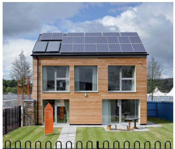
Figure 1: Timber-frame Passivhaus, Ebbw Vale, Wales, using rigid wood fibre insulation on walls both internally and externally
