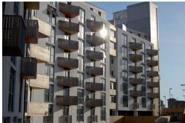
Figure 7: Wood fibre insulation was used on One Brighton as part of a vapour-permeable walling system (Courtesy of Natural Building Technologies)
