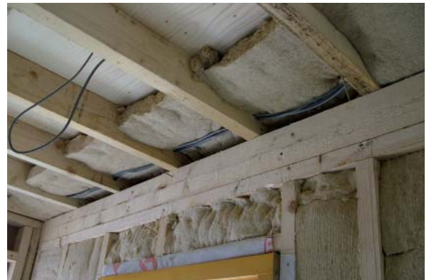
Figure 3: Hemp fibre rolls fitted between studwork (Courtesy of Hemp Technology)
