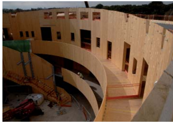
Figure 6: CLT forms solid loadbearing planes, just like masonry walls and concrete slabs, with offsite precut windows and doors
