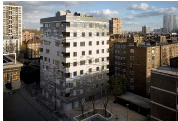
Figure 2: Murray Grove, Hackney, London, is a nine-storey block – CLT panels are used as loadbearing walls and floors (Courtesy of Will Pryce)
