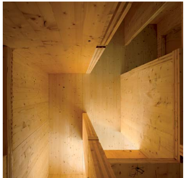
Figure 1: Cross-laminated timber can provide a finished surface as soon as it is installed – installation of future fixtures and fittings is relatively quick and easy (Courtesy of Will Pryce)
