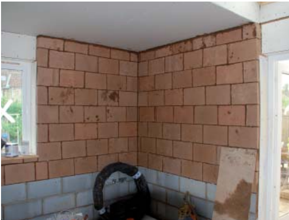
Figure 6: Unfired clay block construction should be used in protected situations, including internal leaves of external walls – this wall is protected by wood fibre insulation and external lime render (Courtesy of University of Bath)
