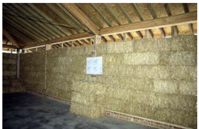
Six courses of straw bale awaiting seventh course (Collins and Beckett)
