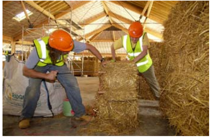
Pinning, tying and cutting of end bales (Collins and Beckett)
