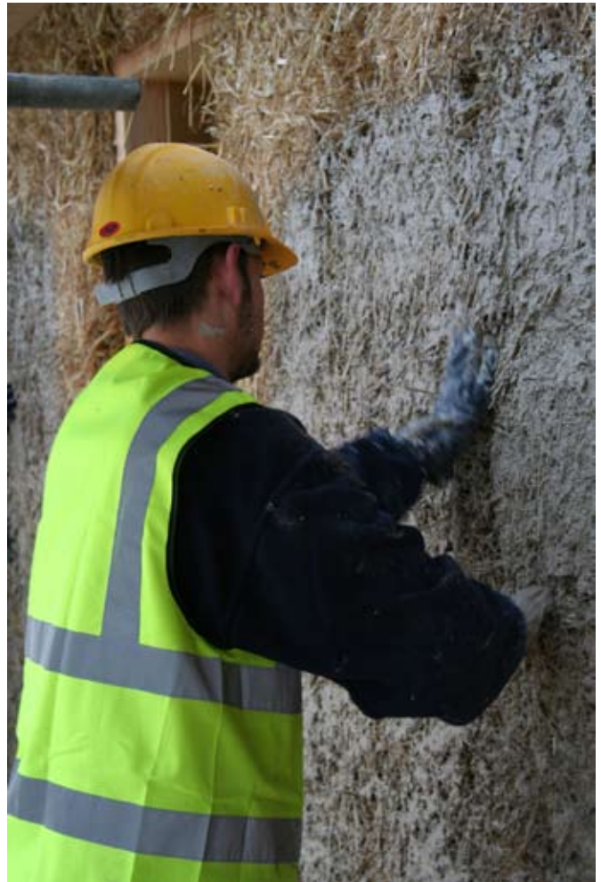
Render being applied to the neat straw face (Collins and Beckett)
