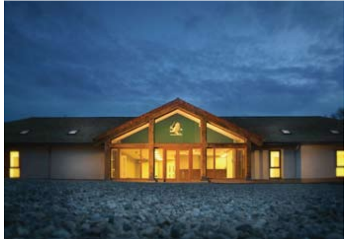
Front facade (Collins and Beckett)
