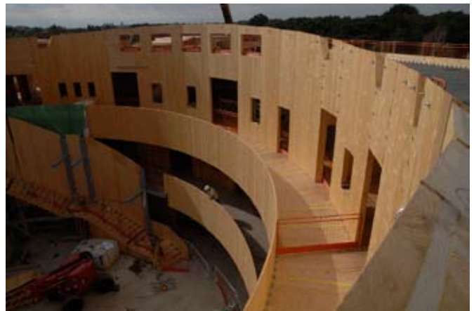
Pre-cut windows and doors (Kier Eastern)
