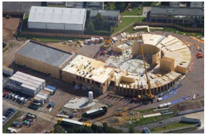
Whole site during construction (Kier Eastern)
