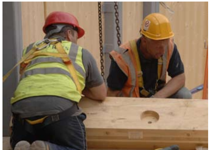
Fitting glu-lam roof beams (Kier Eastern)
