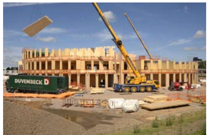
Panels being lifted into place (Kier Eastern)
