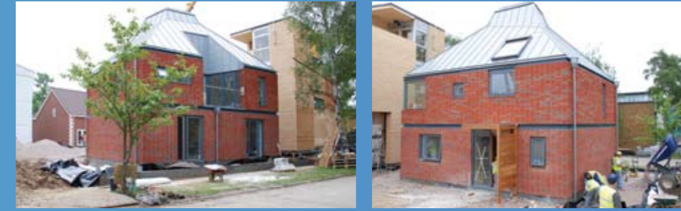
The Hanson EcoHouse™ nearing completion
