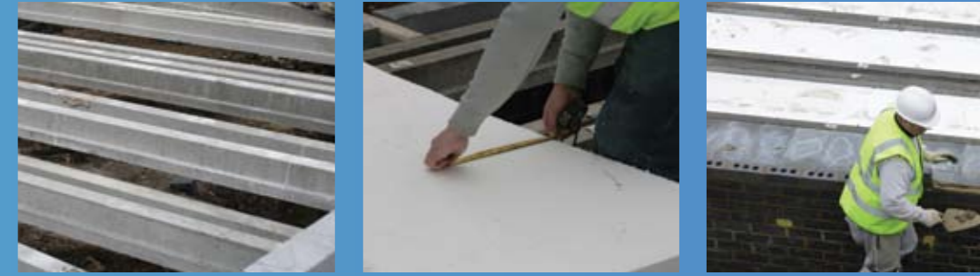
Ground floor installation of Jetfloor
