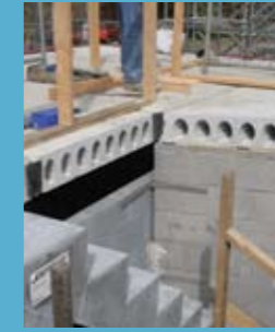
Completion of first floor with prestressed Hollowcore flooring
