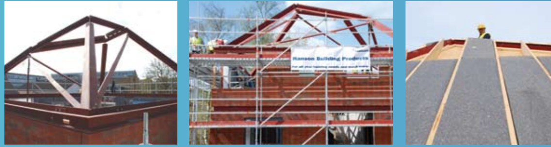
Construction of roof structure
