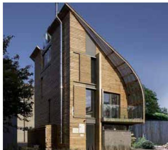
Figure 2 Structurally Insulated Panels (SIPs) were used in the Kingspan 'Lighthouse'
