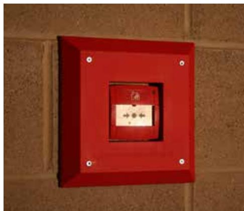
**Figure 8: Protective shielding for manual call points**
