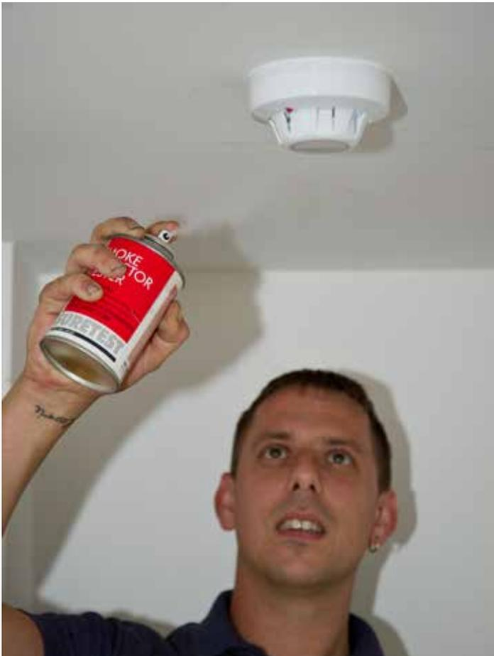
Figure 11 Weekly test of fire detection system
