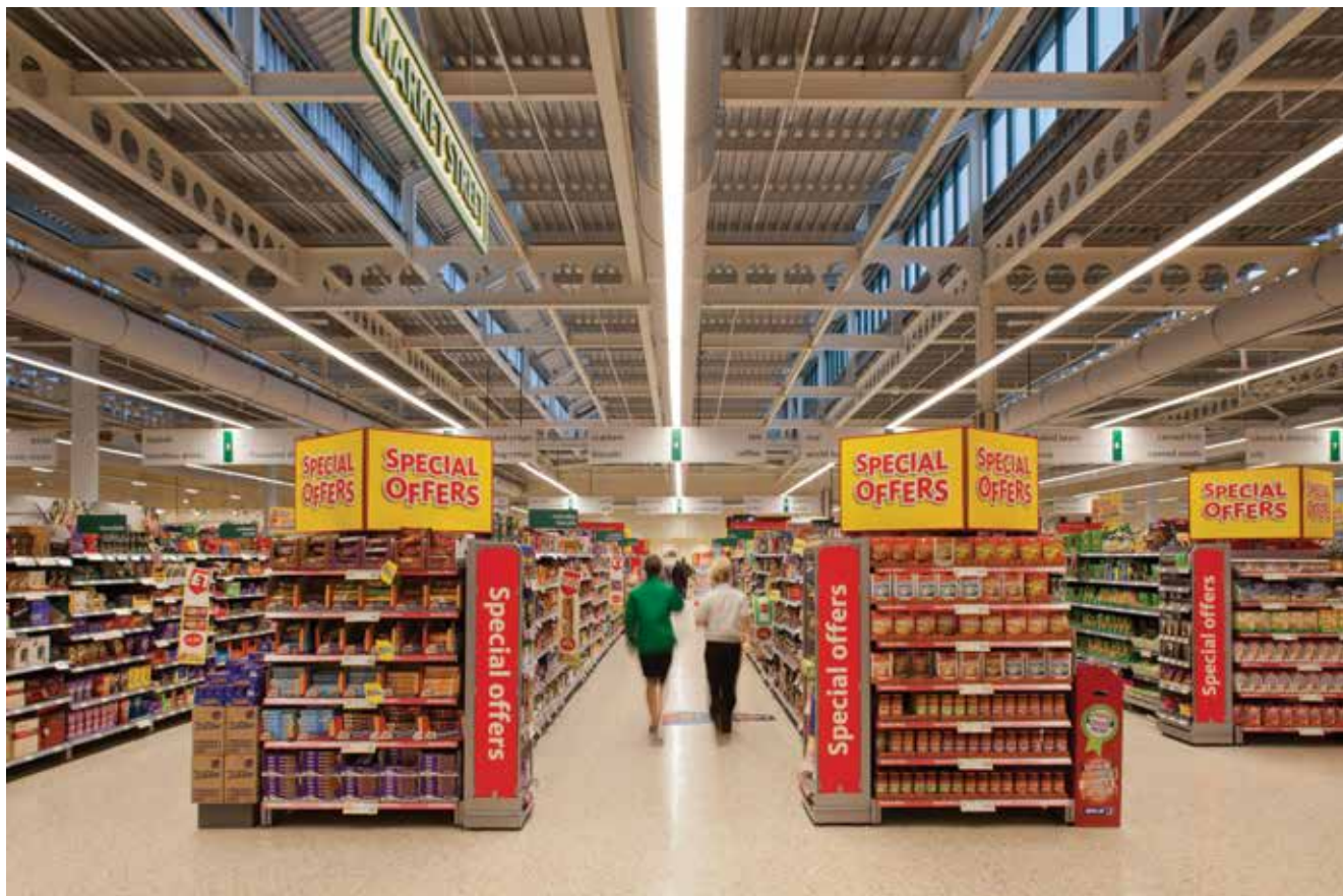
Figure 30: Automatic dimming of electric lighting compensating for daylight variability (© Philips Lighting)
