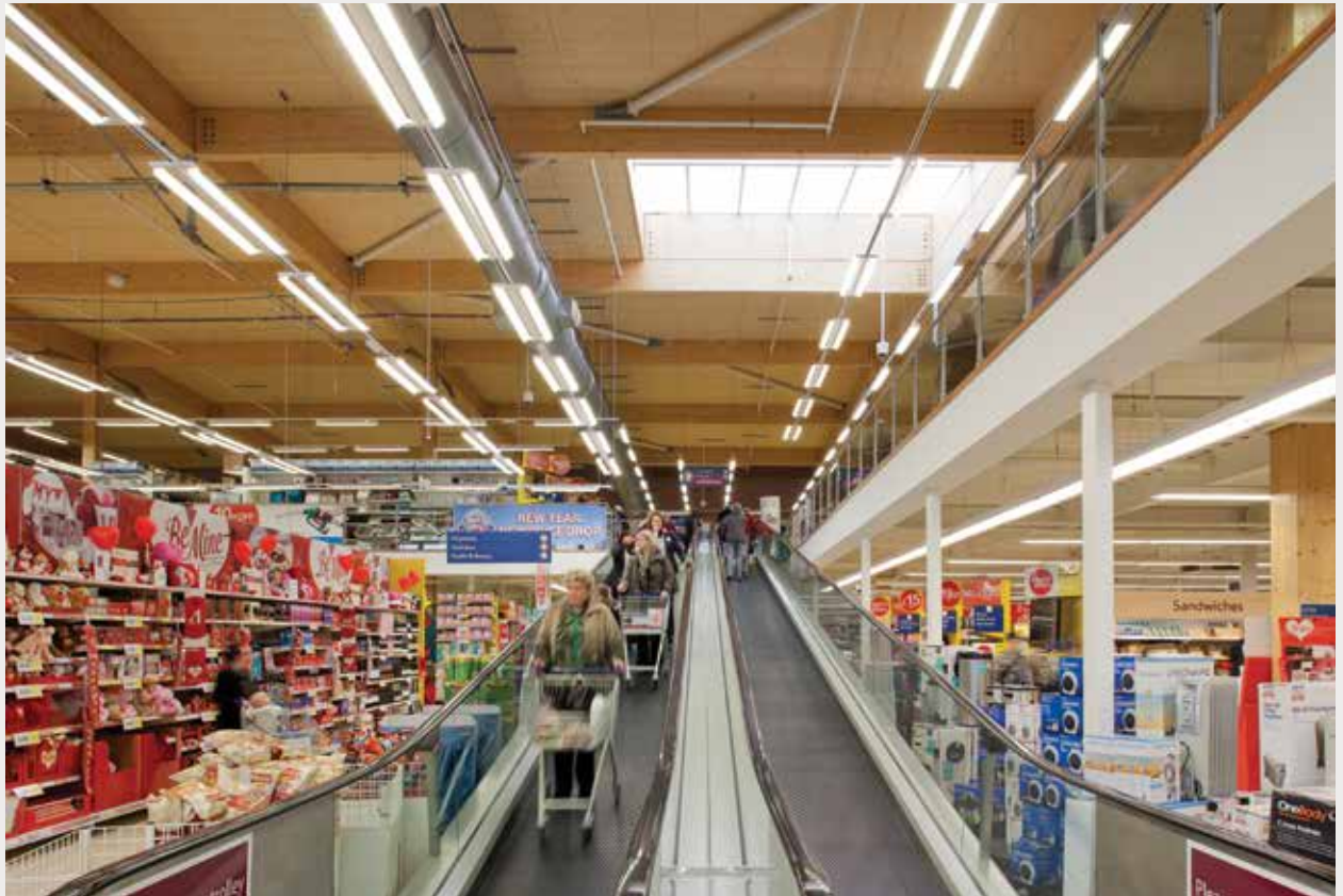
Figure 20: Daylight-based dimmable T5 fluorescent fittings with adjustable reflector and louvre produce the right light output at the level of the merchandise (© Whitecroft Lighting)
