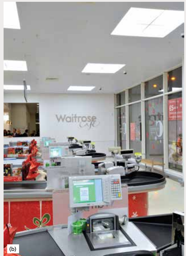
Figure 6: (a) A combination of T5 fluorescent general lighting with metal halide (MH) accent lighting and LED lighting in fridges. (b) Integrated fittings combining daylight from light pipes and electric lamps are used above cashiers (© Waitrose)
