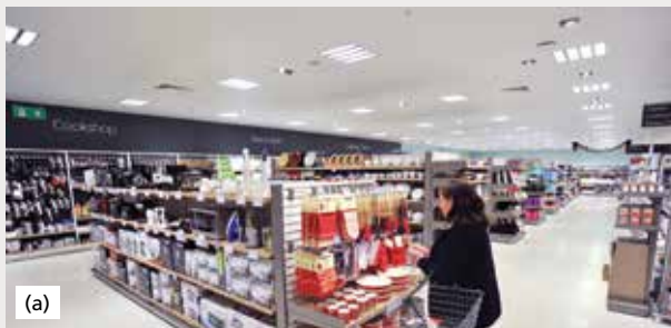
Figure 6: (a) A combination of T5 fluorescent general lighting with metal halide (MH) accent lighting and LED lighting in fridges. (b) Integrated fittings combining daylight from light pipes and electric lamps are used above cashiers (© Waitrose)
