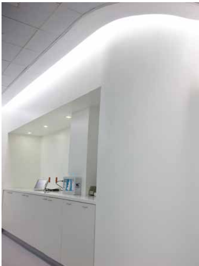
Figure 22: Perimeter lighting by using LEDs in a cove arrangement that can project the light onto the walls or the ceiling (© Philips Lighting)
