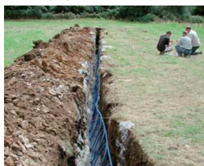
Ground loop trench for ground source heat pump
