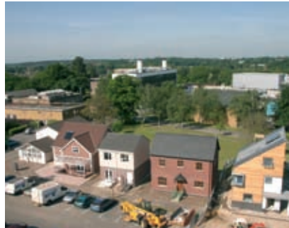
The four demonstration houses at the BRE Innovation park could soon be joined by full-scale education and healthcare buildings
