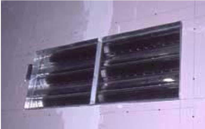
Plate 8. Multi-blade damper mounted in Dry-lined partition
