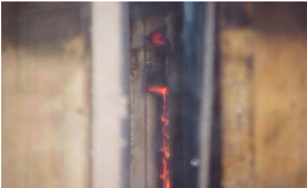
Photograph C9. Showing flames entering the cavity.
