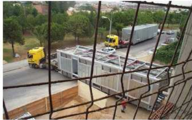
Construction off site
