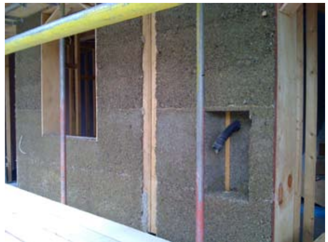
Hemp-lime wall prior to application of render (Glenn Howells)
