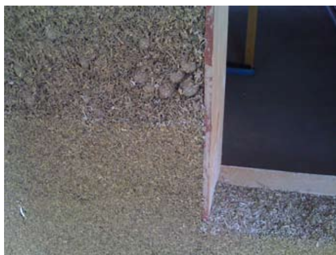
Hemp-lime at window corner (Glenn Howells)
