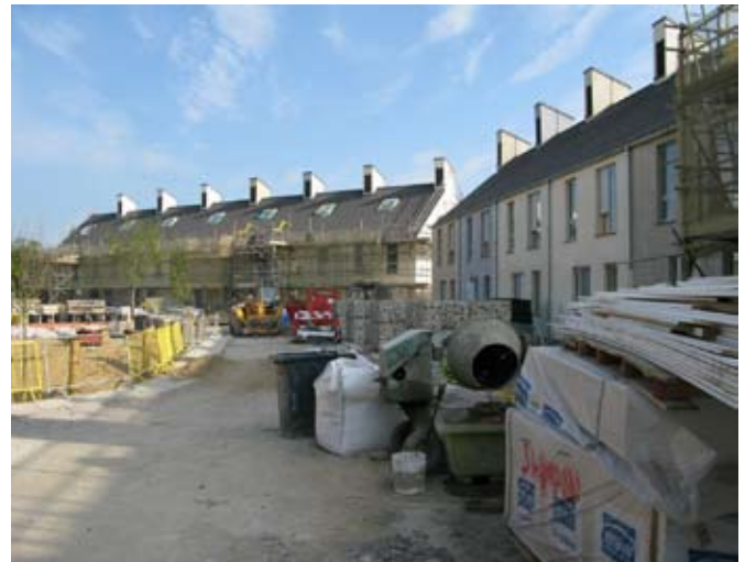
South and west wings just prior to completion (D Black, BRE)
