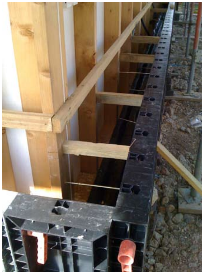
Temporary support for hemp-lime while being cast (Glenn Howells)
