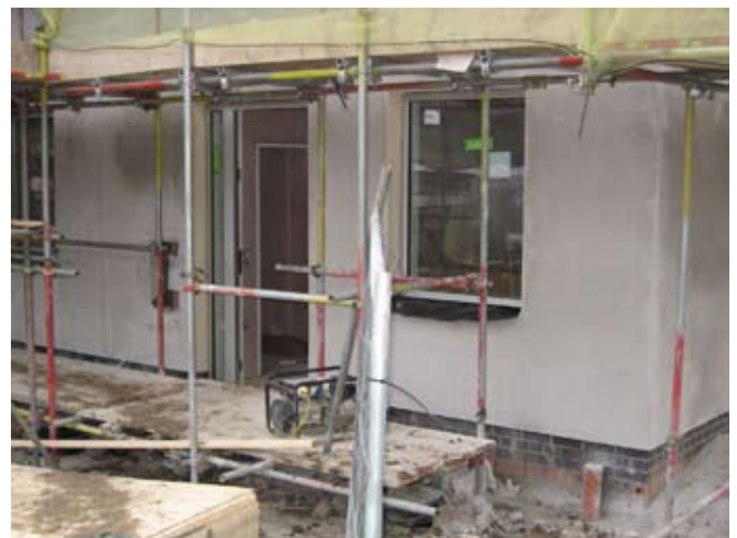
Hemp-lime wall with rendered finish (Glenn Howells)
