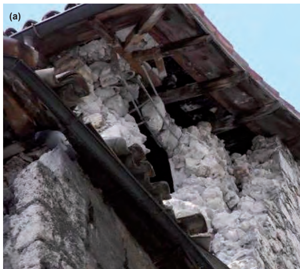
Figure 1: Failures connected to stiffness-based reinforcement (on-site survey, L'Aquila, Italy, May 2009). Detail of reinforced masonry ring beam (a), timber ties (b)
