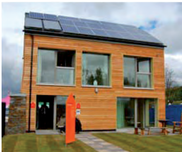
Figure 4: One of two Passivhaus designs being monitored under the TSB Building performance evaluation programme
