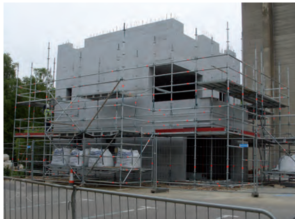
Figure 1: Demonstration units on the BRE Innovation Park, Watford: (a) clay block system superstructure for the Natural House, (b) insulating concrete formwork superstructure for the Creo House
