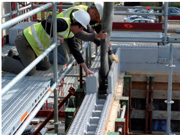
Figure 2: Pouring concrete for the external wall of the Creo House
