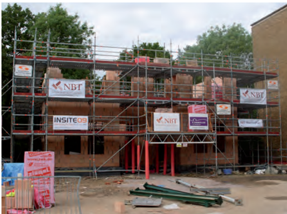
Figure 1: Demonstration units on the BRE Innovation Park, Watford: (a) clay block system superstructure for the Natural House, (b) insulating concrete formwork superstructure for the Creo House
