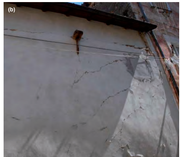
Figure 1: Failures connected to stiffness-based reinforcement (on-site survey, L'Aquila, Italy, May 2009). Detail of reinforced masonry ring beam (a), timber ties (b)
