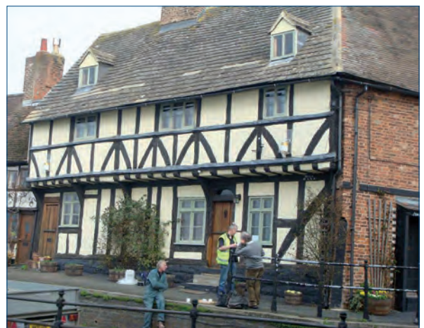
Figure 3: Instrumentation on 1 Mill Bank, Tewkesbury
