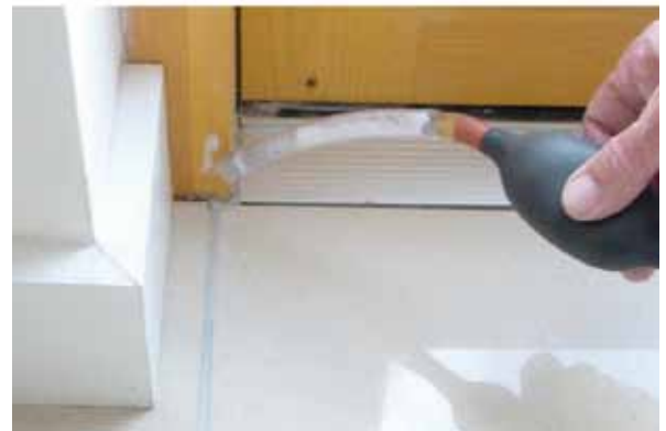
Figure 2: Testing for the air tightness in dwellings built to Passivhaus standard
