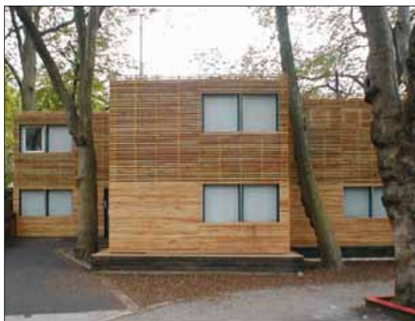
Figure 1: Modular buildings built near to trees supported on removable steel screw piles, as an alternative to permanent concrete foundations Courtesy of ScrewFast Foundations
