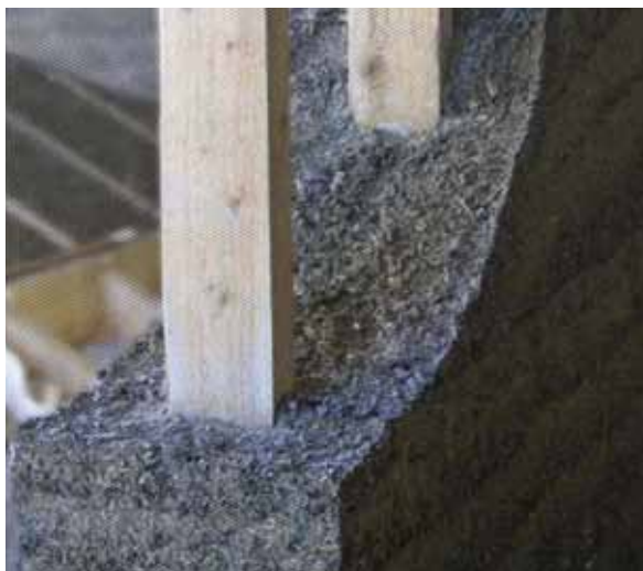
Figure 1: Hemp–lime cast around a timber primary structure Courtesy of Lime Technology 2008
