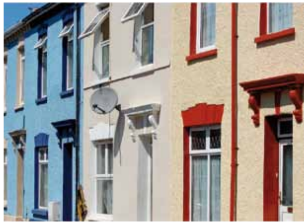
Figure 4: The UK has many buildings with thick stone walls that will be addressed in the SUSREF project
